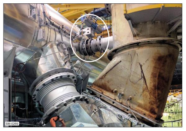
Figure 2-23: Exhaust gas waste gate (EWG) installation
